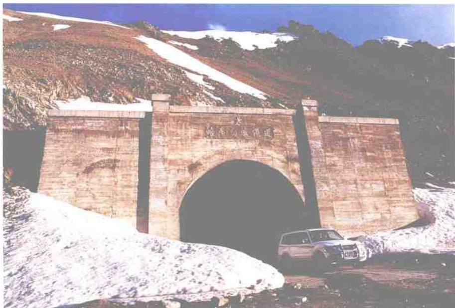
独库公路哈希勒根隧道 Haxilegeng Tunnel of Du-Ku Highway
