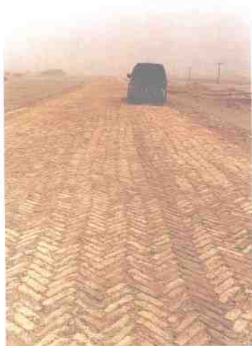
218国道的红砖路 The No.218 National Highway Paved with Red-Brick
