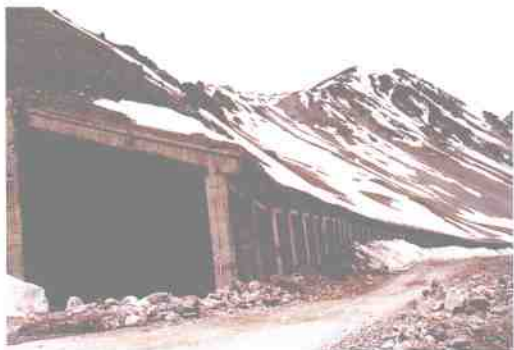
独库公路防雪走廊 The Snow-blocking Corridor along Du-Ku Highway
